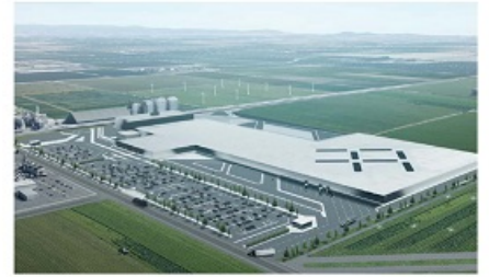
2 1.1 MILLION SQUARE FOOT MANUFACTURING FACILITY IN HANFORD, CA
